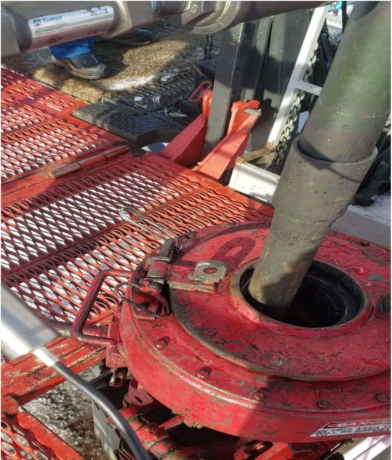
Figure 2.5 – Tubing set in air slips with power tongs over top.
